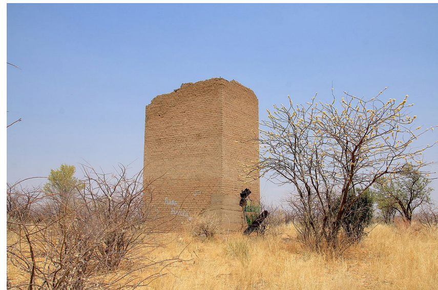
Abspannpunkt eines Funkmastens in Windhoek, 2024. Guy-wire attachment point of an antenna in Windhoek, 2024. Foto Photo: Frederike Moormann
